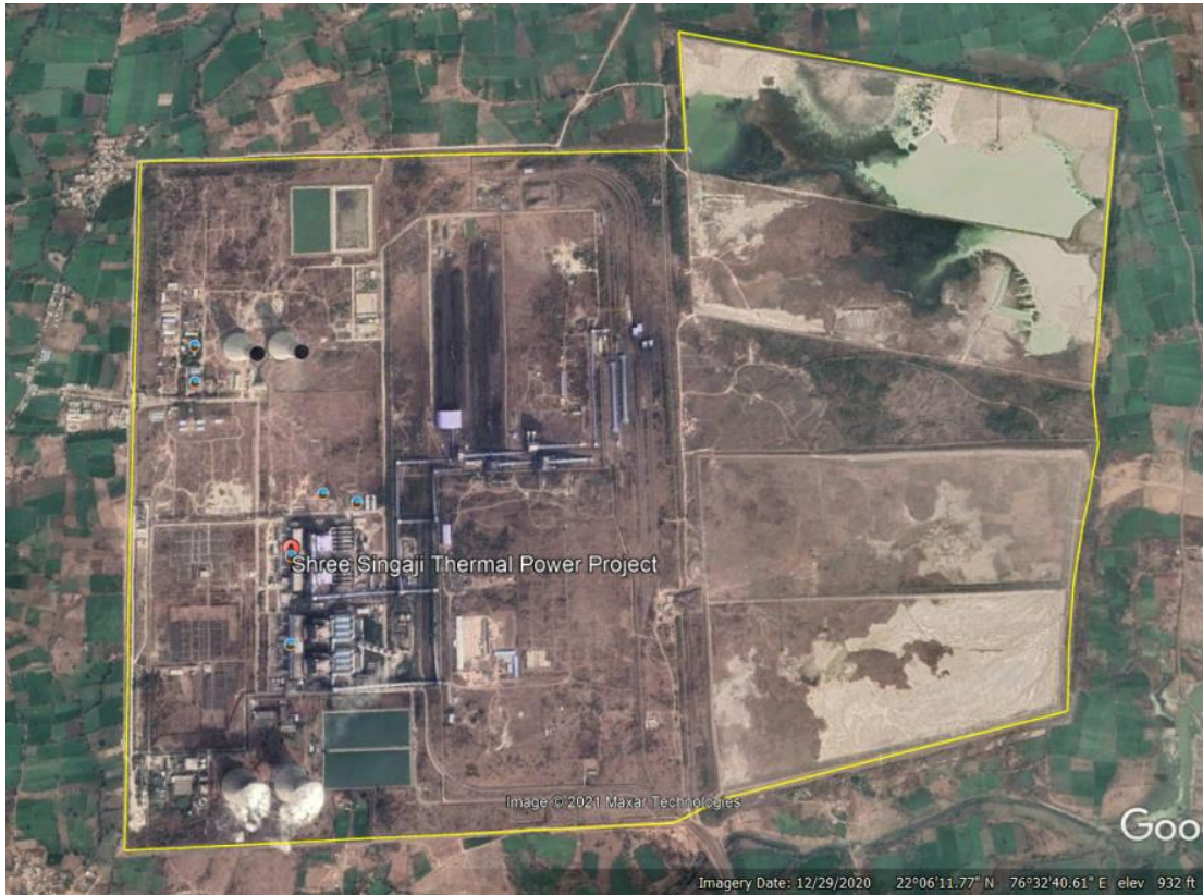
Figure 11: Shri Singaji Thermal Power Project (Area 10.3 sqkm)
