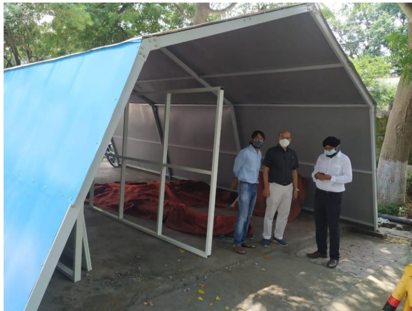
Figure 2: Erection of Makeshift Clinic under progress
