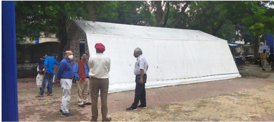
Figure 3: Inspection of erected Makeshift Clinic
