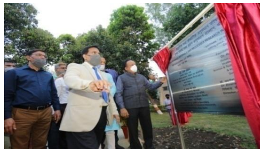
Laying the Foundation Stone of CSIR-AMPRI Bamboo Composite Structure ‘BAITHAK’
