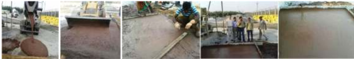
Laying of road at site utilizing JSPL fly ash
