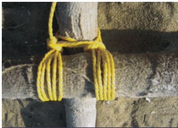
Method of tying the reinforced bamboo
