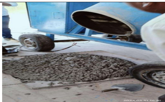
Mixing and Development of Geopolymeric Concrete
