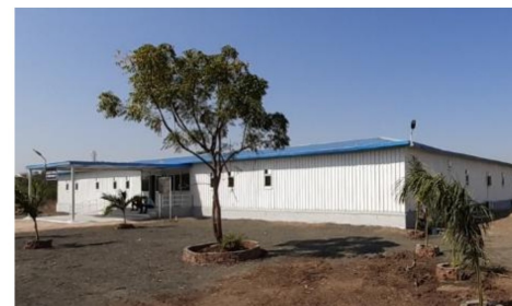
30 Bed hospital erected with makeshift technology at Nandurbar
