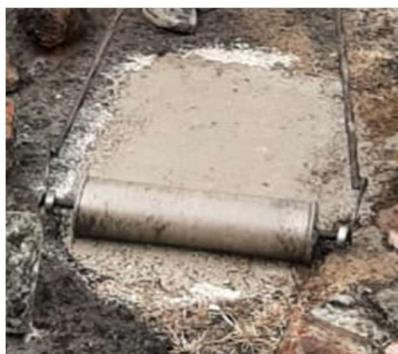
Patching on Cement Concrete Surface
