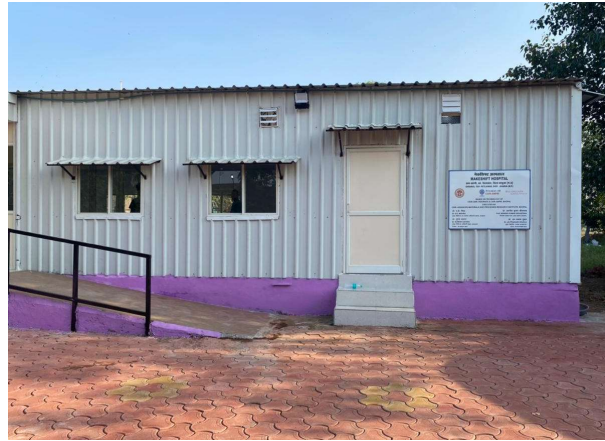
Ramp with railing for stretcher, patients; emergency exit door in the general ward
