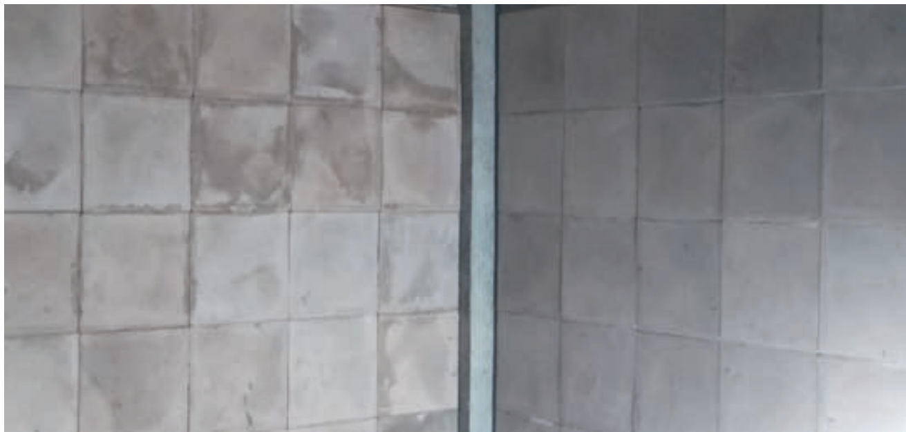
Figure 23 Joint free X-ray shielding tiles that are paved on the wall of X-ray attenuation facility developed at CSIR-AMPRI, Bhopal.
