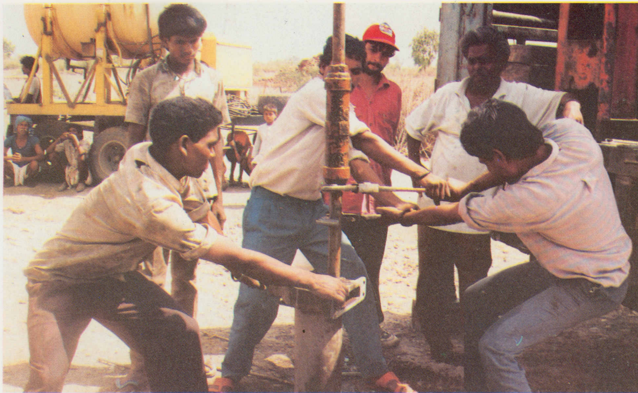
Dismantling hand pipe line alongwith cylinder for chemical hydrofracturing
