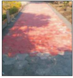
Demonstration of Advanced LSA based Geopolymer Concrete Paver Blocks in front of workshop at CSIR-AMPRI
