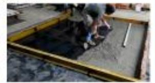
Preparation of mold and pouring bottom layer of concrete
