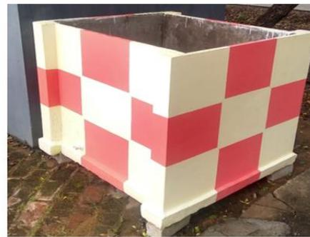
Water Tank with Pre-cast concrete panels
