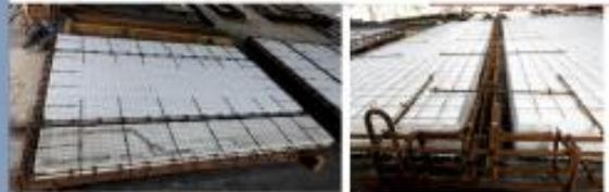
Preparation of Reinforcement Cages in the EPS Panel
