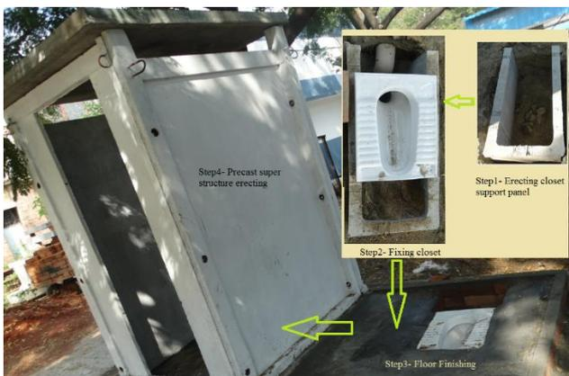
Type4- Single Toilet Units (Dry joint mechanism)
