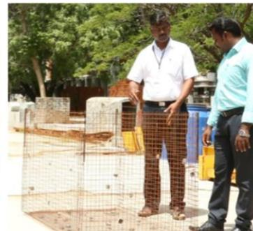
**Reinforcement : Weld mesh of size 25mm x 25mm with 2.3mm dia. wires**
